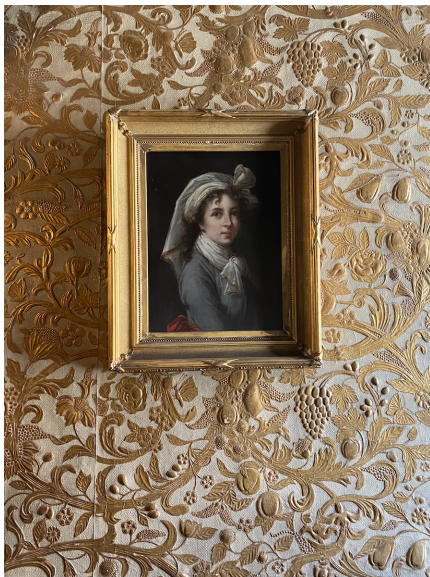
Fig. 2. Japanese leather wallpaper in the Gibson House Museum. A crease towards the left side of the photo shows how the panels of the wallpaper come together. A framed painting was also placed on top of the wallpaper.
